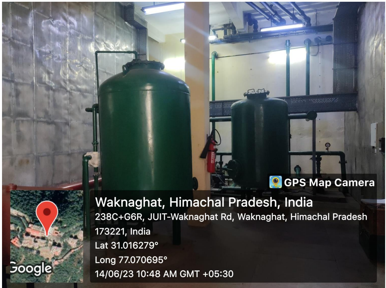
Figure 12 – Raw water Polishing system before pumping to overhead tanks
