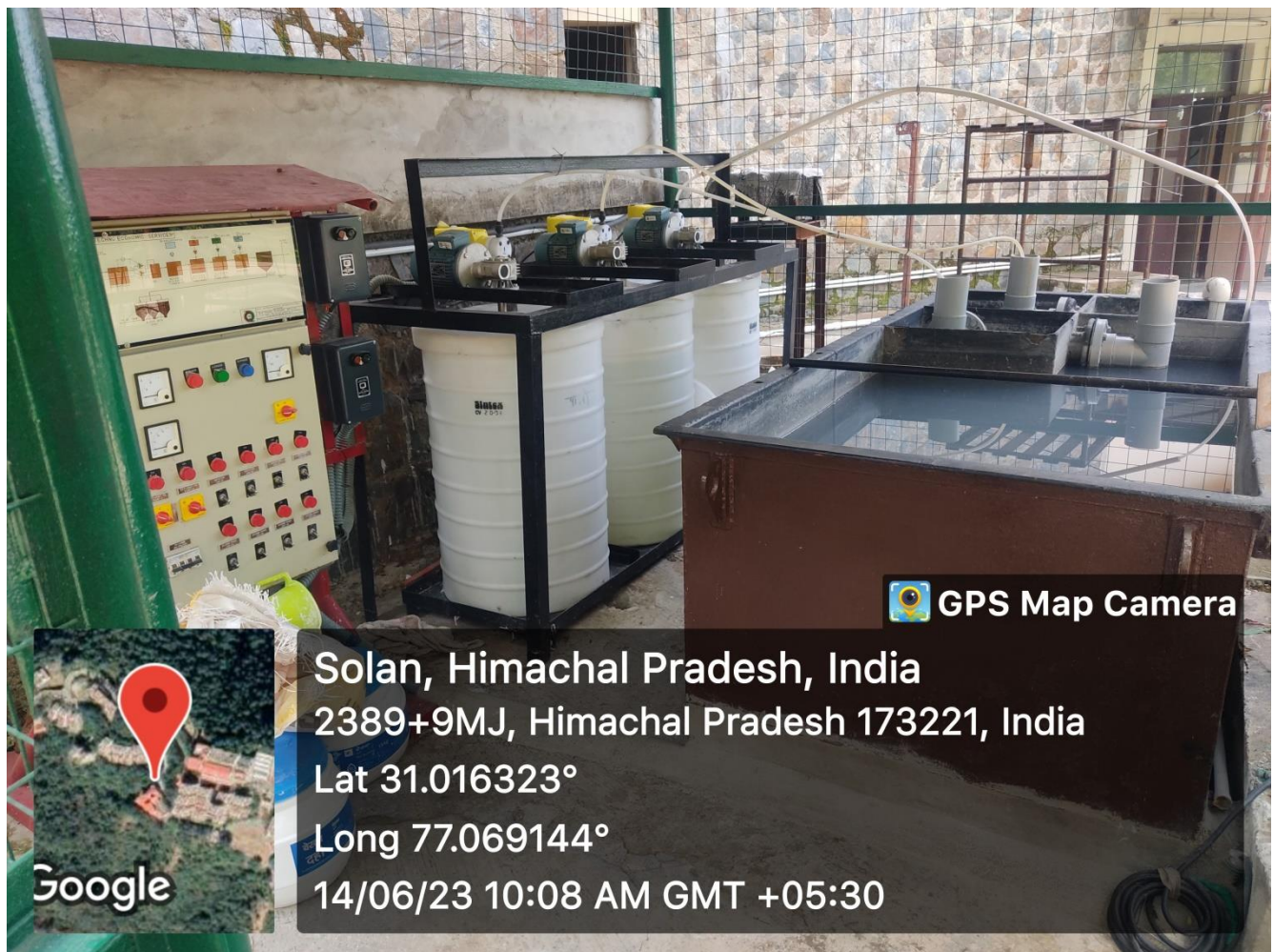
Figure 15 - ETP for laundry waste water
