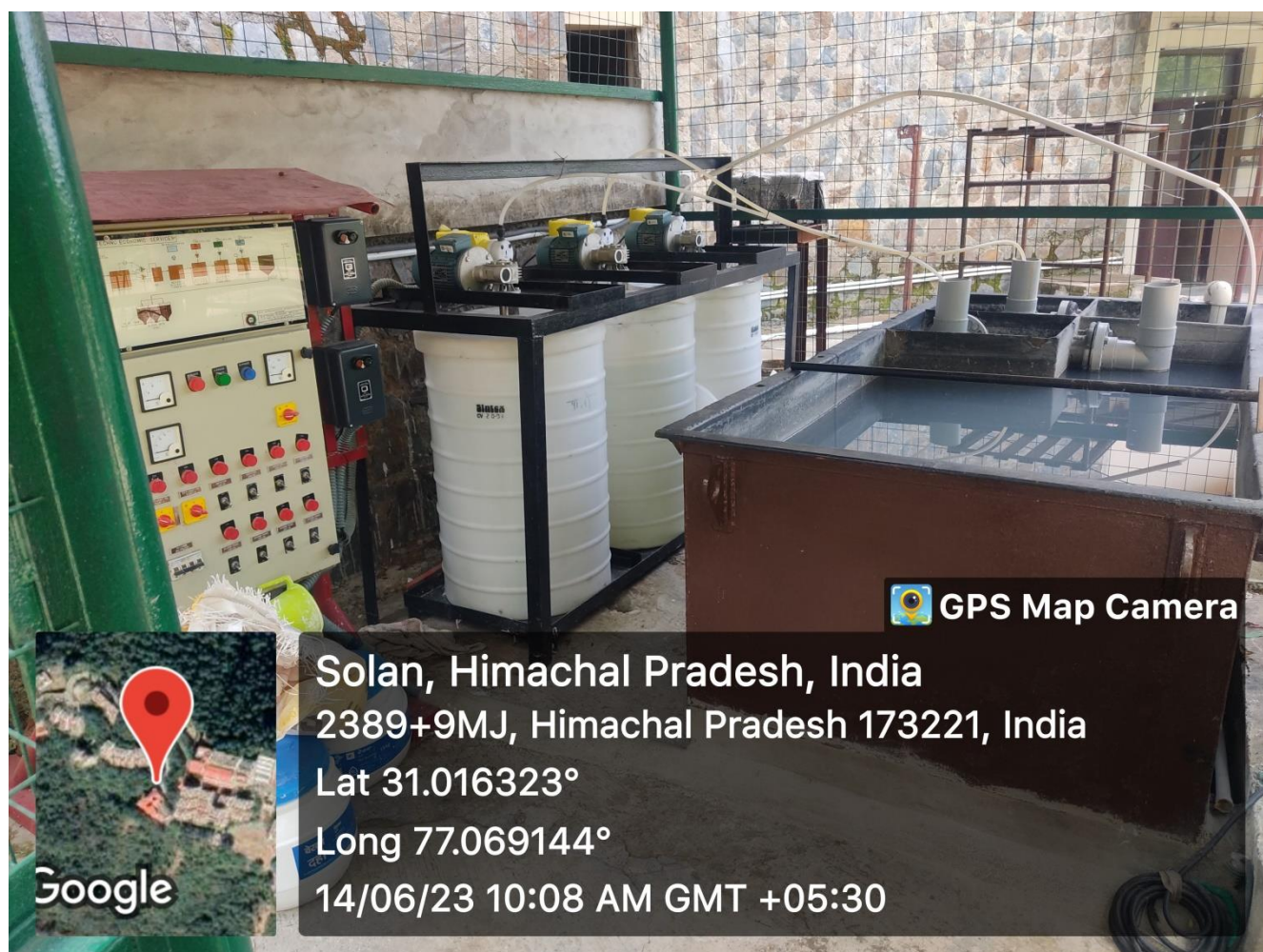
Figure 25 - ETP for Laundry waste water
